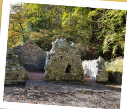
Conserved historic remains of the Gunpowder Works, Afon Mellte
